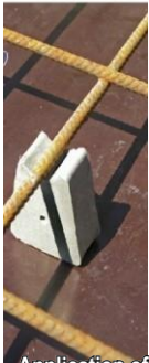
Application of Footing Cover Block
